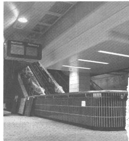
(Below right). Experimental station finishes installed to evaluate design, colour schemes, and material prior to completion at Museum Station site.
