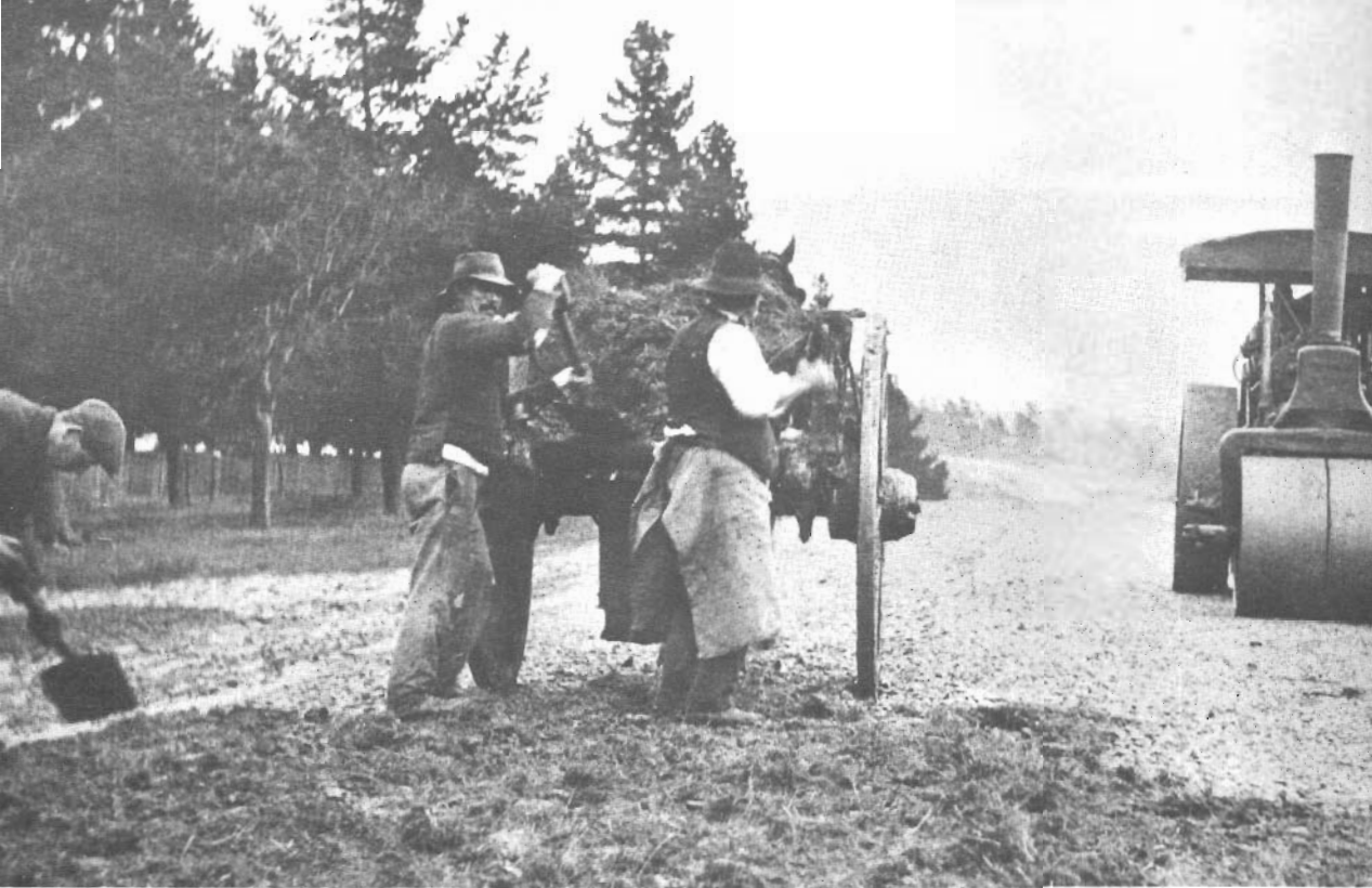
Dandenong Road in 1913. A form of road construction using metal, soil, weeds, and grass to provide a surface.
