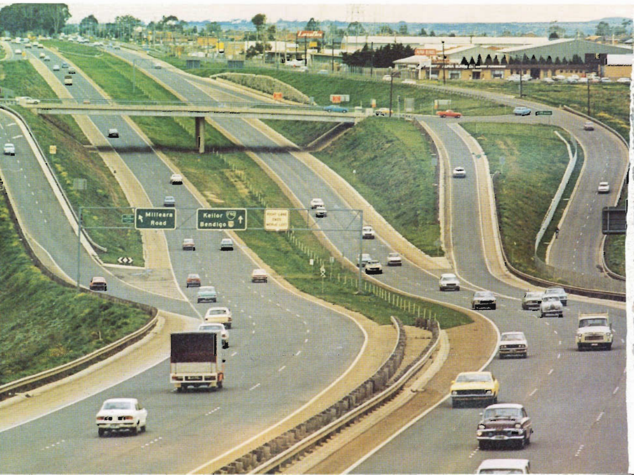
A section of the Calder Freeway passing through the City of Keilor. Country Roads Board
